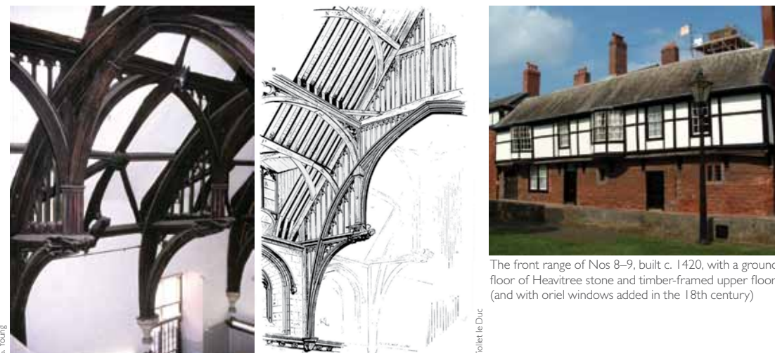
Detail of the Law Library roof, No. 8. The Close (left). This magnificent roof was built about 1420. Its design is very clearly derived from the greatest hall roof of medieval England that over the great hall of the Palace of Westminster, constructed in 1395–9 (right).
