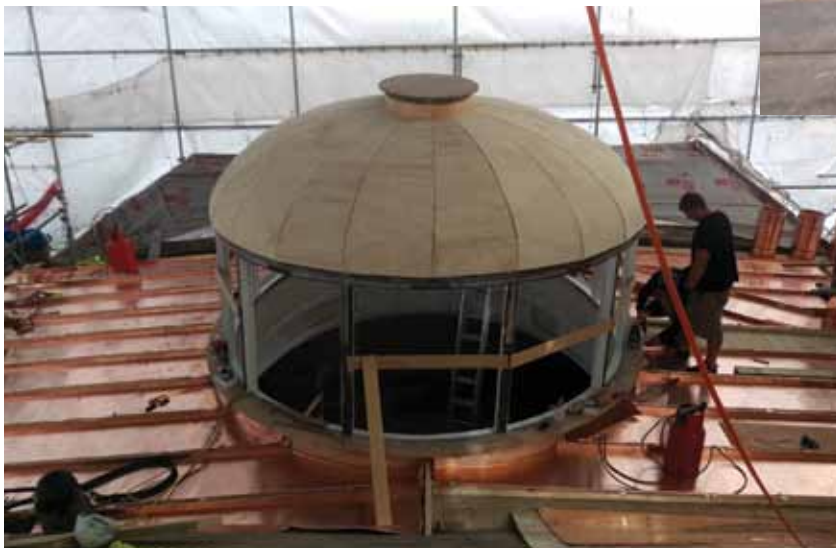
The copper cladding is fitted, September 2016
