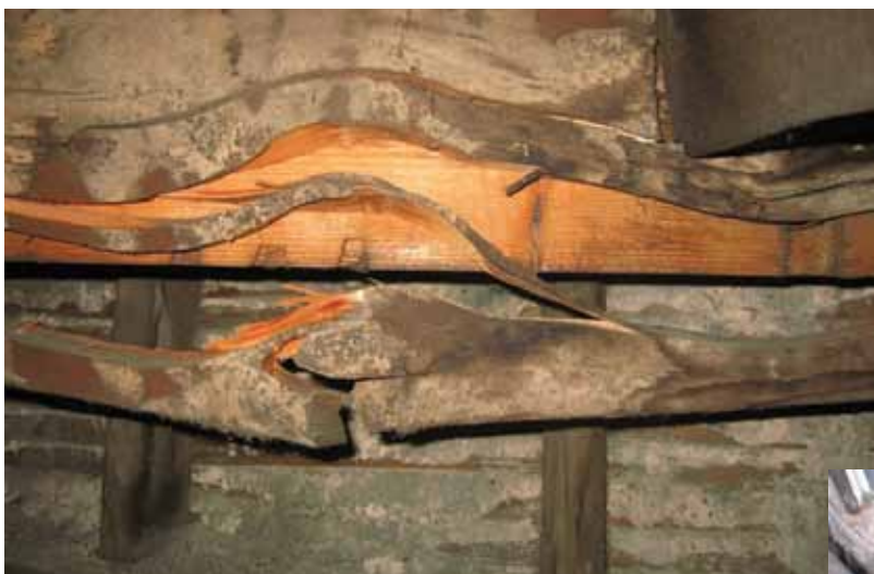
Failed timbers beneath the Inner Library cupola, 2014
