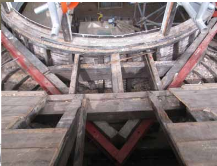
Templated steel encases the failed timbers, June 2016
